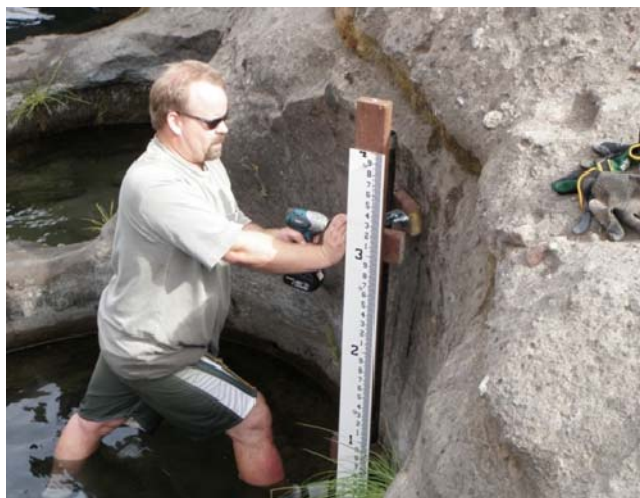
Figure 8. Installation of Staff Gauge along Mill Creek
