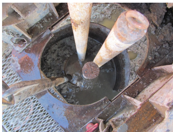
Figure 12. Adding Grout Seal during Construction of MW-CSU-1
