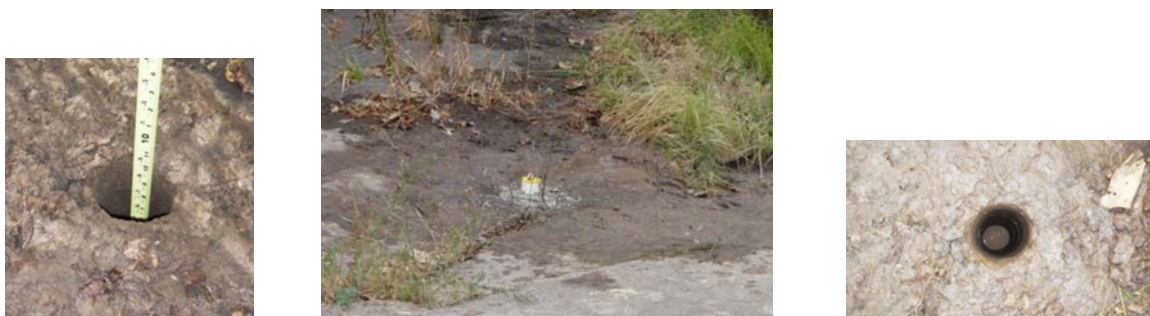
Figure 10. Temperature Gradient Well Installation along Mill Creek
