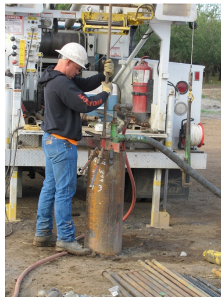
Figure 13. Development of MW-CSU-1
