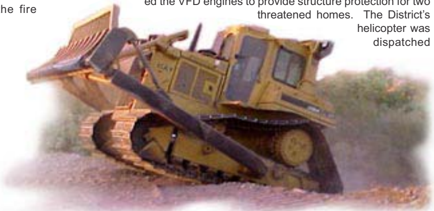
USFWS Dozer Performing Initial Attack on Hippy Fire; Yuma, AZ in 2002 Courtesy of Wildlandfire.com
